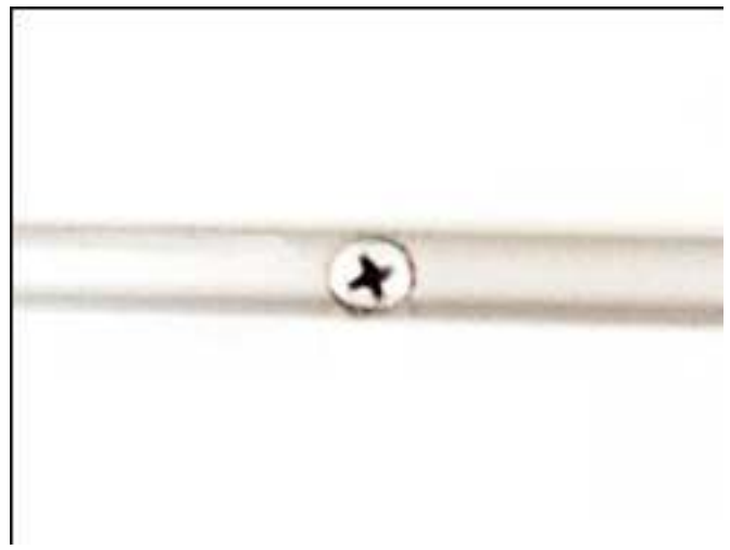
STEP 5 – SCREW HEAD FLUSH
